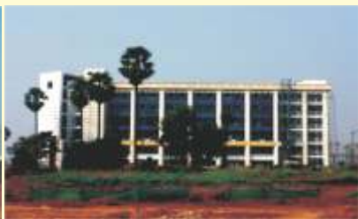
Academic Block No- 03 Dept. of Mechanical, Electrical & Computer Sc. Engg.
